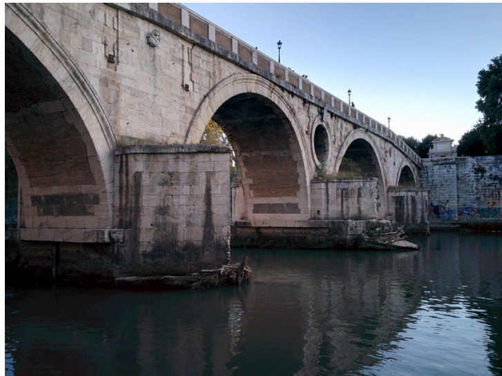
Fig. 8. Ponte Sisto, the cutwaters. Photo: Marco Mininni
