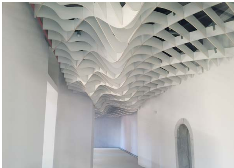
Fig. 5. Installation of the ceiling.
