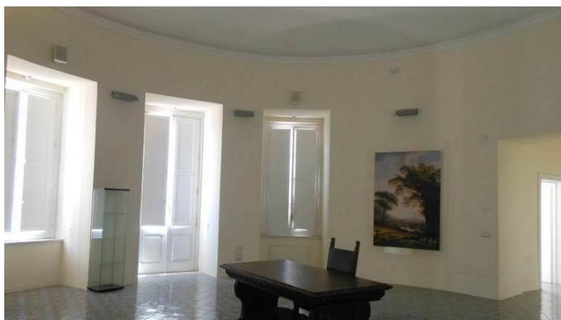
Fig. 4 Image of the circular room on the first floor.
